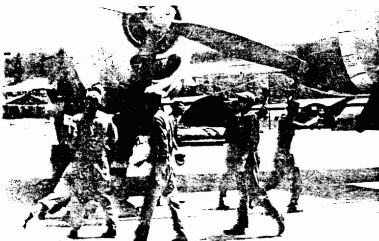
Pulling props through prior to engine start
